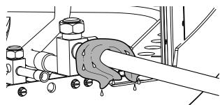
Figure 16: Cool the Joint After Brazing
